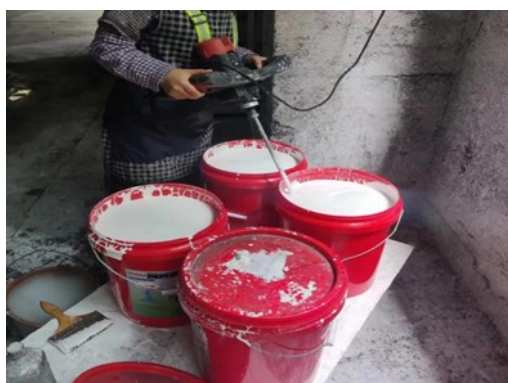
Figure 9. Mixing of coating material in open containers (left) and coating material brushing operation (right).
