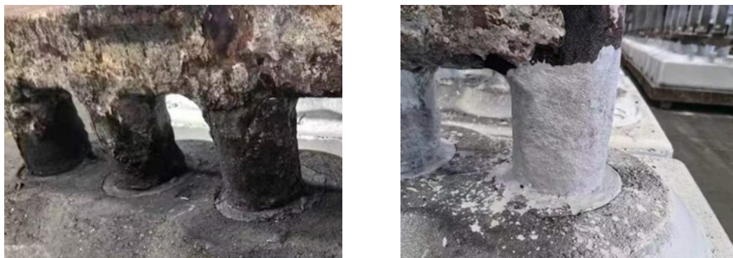
Figure 10. Stubs with materials but not coated yet (left) and coated stubs right.
